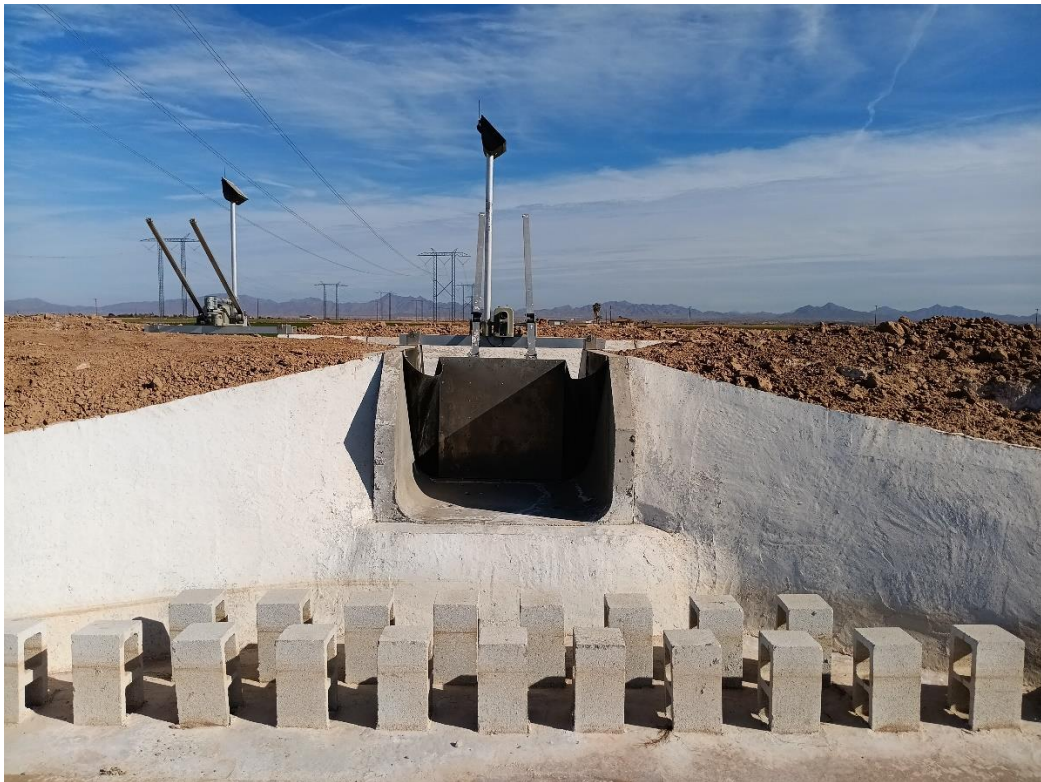
Figure 3 BayDrive actuation for border check systems
